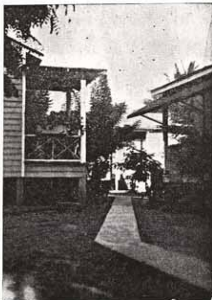
St. John's Day School Buildings. Two more buildings are located in the rear, one of which can be seen. The other is a garage converted into a school room.
