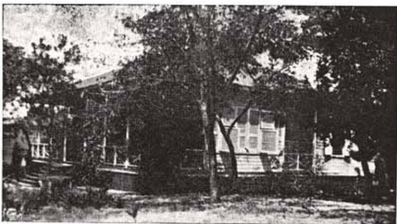
St. Catherine's Training School, building and grounds, Santurce, where new centralized church group is to be located.
